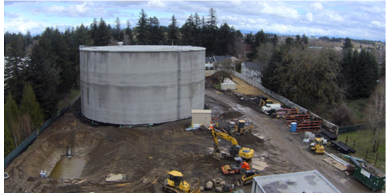
Cascade Reservoir 2. Photo taken April 07, 2023
