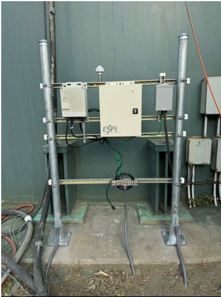
Photo: AMI Collector at Cascade Reservoir #1
